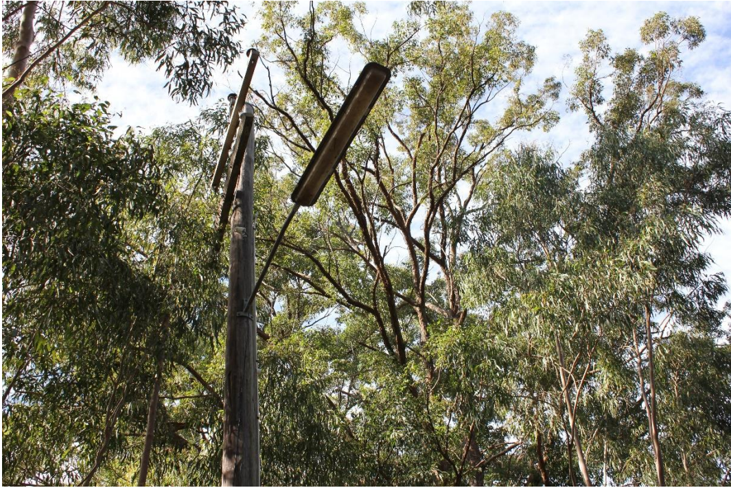
13. Retained timber telegraph pole with attached street light along the former bitumen roads within Precinct 3. Source: TKD Architects, 2022
